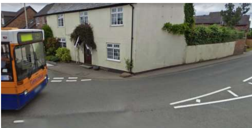
Photograph showing the footpath adjacent to 1 Church Street, Sapcote adjacent to the B669 (southern side). Here the footpath is less than 1.0 metre wide and reduces down to nothing on the junction.
